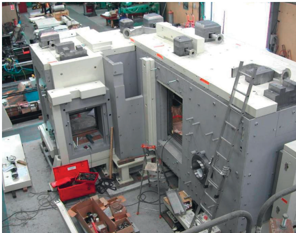
Fig 84. Construction of shielded cells for the VERDON experimental device at the STAR underground laboratory.
