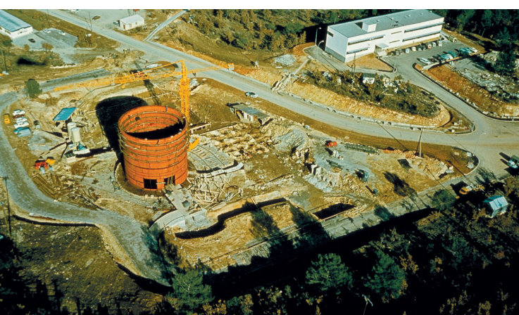
Fig. 47. Construction of the MASURCA reactor.
